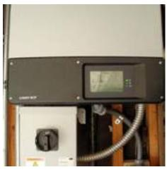
This handy product produces 1500 watts of 120 volts AC and can provide 12.5 amps if grid power goes out and the sun is still shining. I need 6.5 amps even though the refrigerator-freezer operates on a 20% duty cycle (draws 6.5 amps 20 percent of the time when the compressor is running), so the secure power from the inverter works just fine during sunny days. Figure 2 shows the configuration chosen for this application.
